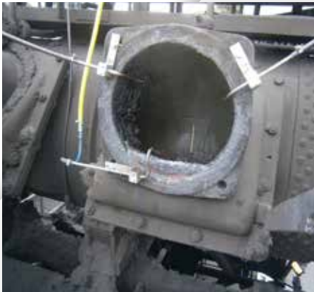
Cast iron conduct of coke plant (FAR 3556)
