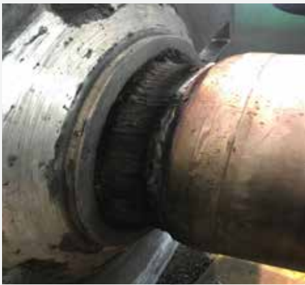
Drawing shaft repaired (FAR 26519)
