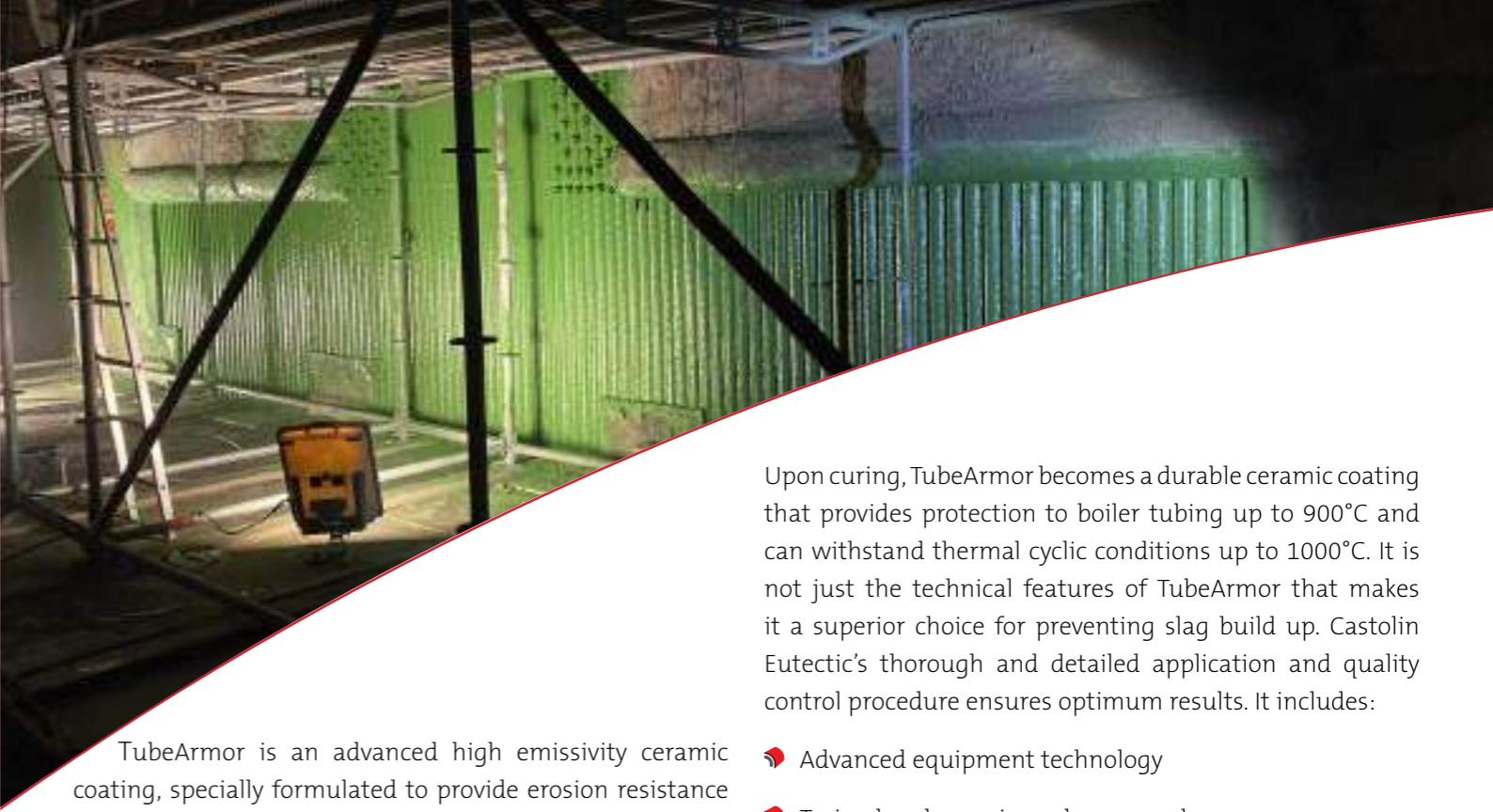
TubeArmor is an advanced high emissivity ceramic coating, specially formulated to provide erosion resistance and corrosion protection while increasing heat transfer and thermal efficiency. The coating is a high solids system which is applied as a stand-alone dry film at thicknesses up to 0.5 mm. It is thermally conductive and bonds extremely well to properly prepared steel substrates. TubeArmor is also applied over our ChromeClad thermal spray coatings.
